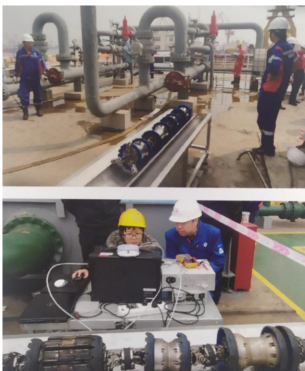
Fig. 4. Implementation of the technology for detecting magnetic flux leaks in pipelines
