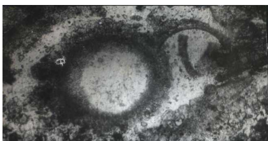
Fig. 1. Photograph of a section of a reinforced concrete sample with traces of carbonation of the protective layer of concrete near the reinforcement. x10. (Photo by the authors).
